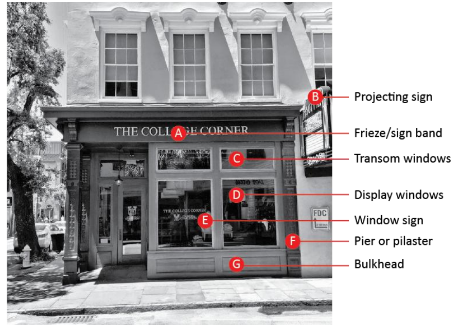
Figure 49 Parts of a traditional Storefront
