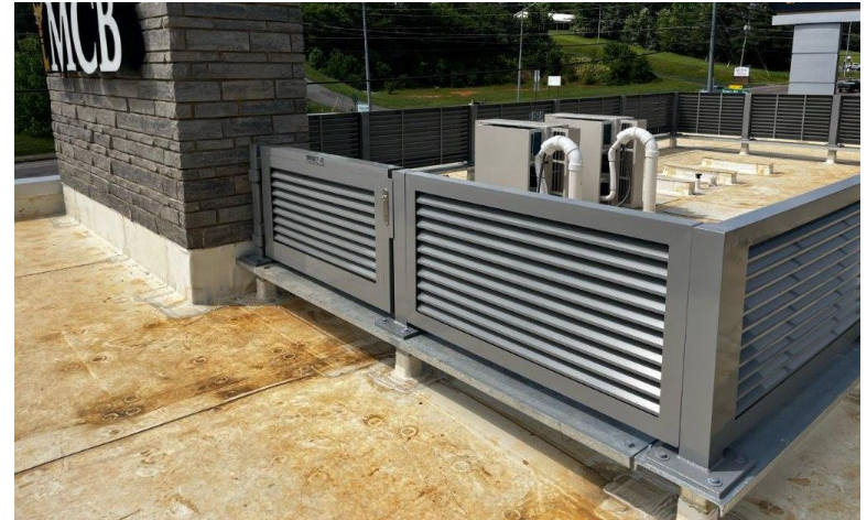
Figure 12 Screening may be necessary when location on the roof is not sufficient to obscure views of mechanical units from public view.
