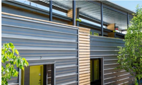
Figure 21 Standing seam metal siding
