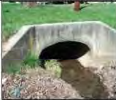
Elliptical RCP; Measure both horizontal and vertical diameters.
