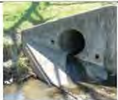
CMP round pipe with two weep holes at bridge crossing. (Don't mark weep holes)
