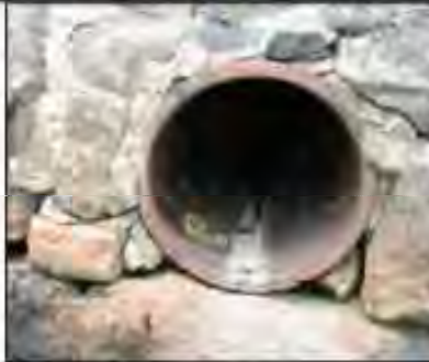
Staining at the base of the outfall may indicate a persistent, intermittent discharge.
