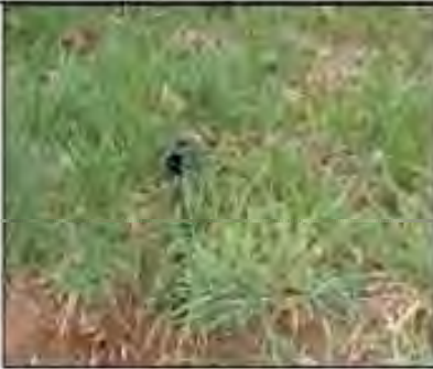
Small diameter (<2") HDPE; Often a sump pump (legal), or may be used to discharge laundry water (illicit).
