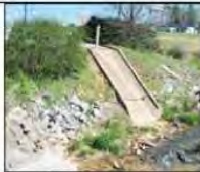
Open channel "chute" from commercial parking lot; Very unlikely illicit discharge. Mark, but do not return to sample (unless there is an obvious problem).
