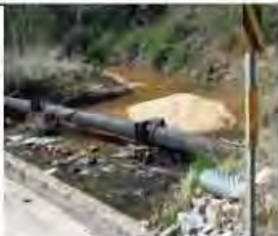
CMP outfall; Crews should also note upstream sewer crossing.
