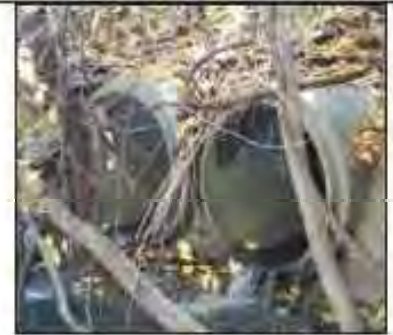
Double RCP round pipes; Mark as separate outfalls unless known to connect immediately up-pipe
