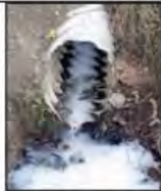
Paint Color: White; Severity: 3 Turbidity: 3
