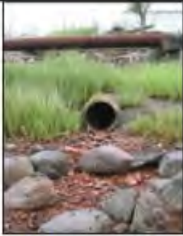
Reddish staining on the rocks below this outfall indicate high iron concentrations.
