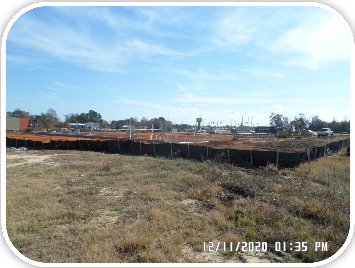
Example of construction site after corrective action
