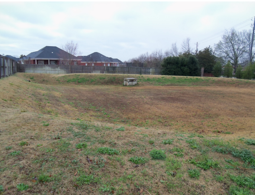
A well maintained detention pond
