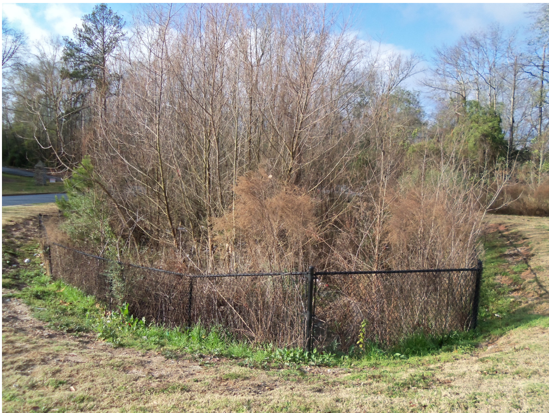
Detention pond in need of maintenance
