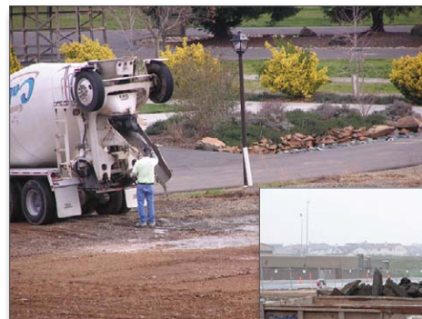
Figure 1. Chute washwater being dumped on the ground
